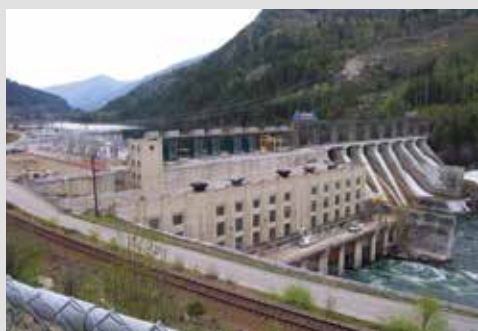
BC Hydro's Bridge River Complex, Canada
