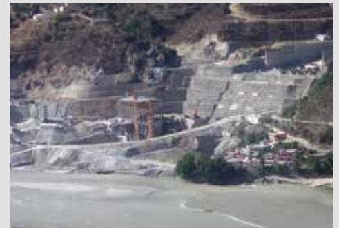
Alakanada Dam, India
