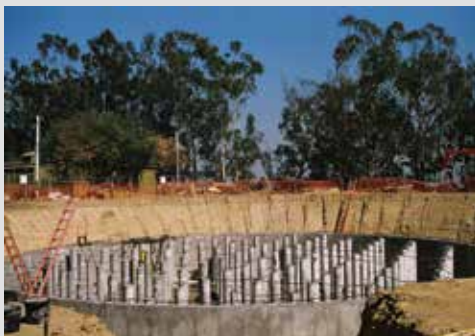
TreePeople Center Cistern, USA
