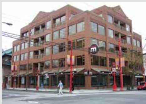
Channel M Building, Vancouver, Canada
