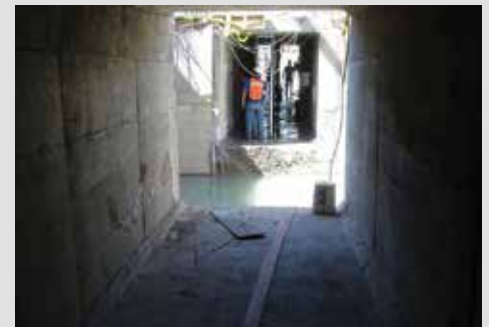
Ensenada International Terminal Tunnel, Mexico
