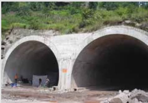
Yunnan Shuima Tunnels, China
